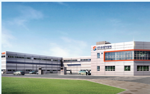
Construction of a factory for Yuwon EM Tech Co., Ltd. in Geochang
