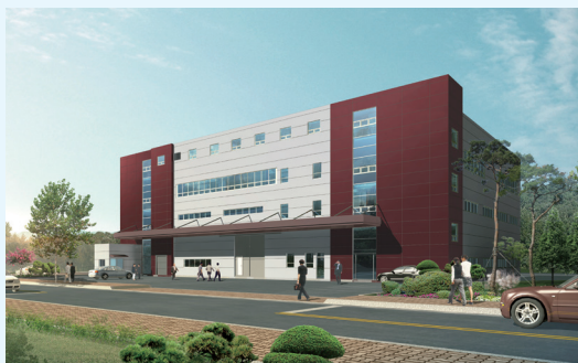
Construction of a factory forTECHEN Co., Ltd.
