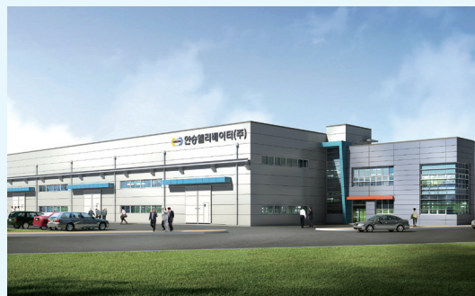
Construction of a factory for Anseong Elevator Co., Ltd. at Geochang General Industrial Complex
