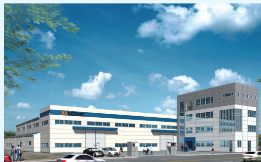
Construction of a factory for Modun Net Co., Ltd. at The 5thSeongseoHigh-tech Industrial Complex
