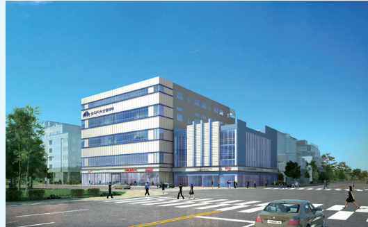
Construction of a factory for Moda Knowledge Industrial Center Co., Ltd. - 1
