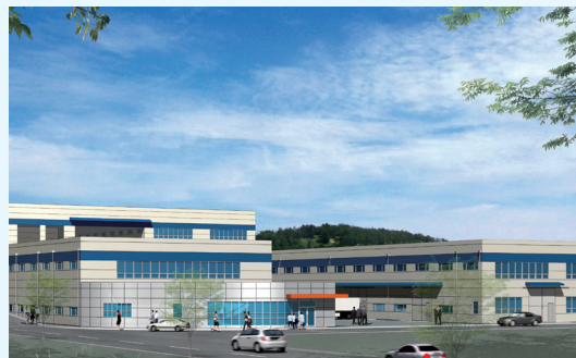
Construction of Knowledge Industrial Center for Vision D&C Co., Ltd.
