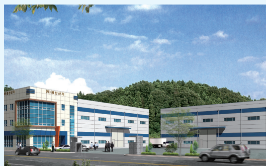
Construction of a factory for Gumsan Sanki Co., Ltd. in Geochang
