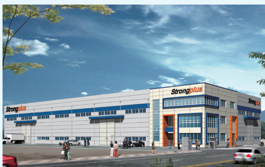
Construction of a factory for Strong Plus Co., Ltd. at Geochang General Industrial Complex
